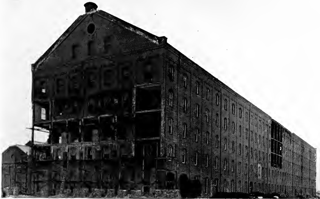
A. Spreckels sugar mill, near Salinas. Entire building buckled. Looking southeast. R. L. H.
